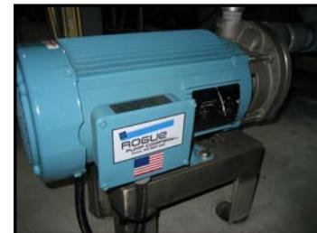
RPC determined that replacing the existing aeration system with a new AISI 316 stainless steel **MAX RGT™** regenerative turbine pump, a superior upgraded DAF was possible. The new system entailed the pump, control valves, gauges and schedule 80 PVC piping. All were to be positioned conveniently below the DAF adjacent to the effluent chamber. The design recycled effluent water through the pump and would achieve saturation it in a single pass.
