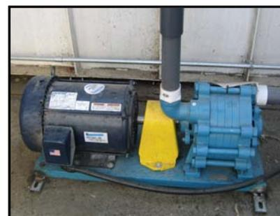
With the new pump technology a superior upgraded DAF would be the result. The new system entailed the pump, control valves, gauges and PVC piping. All were to be positioned conveniently beside the DAF adjacent to the effluent and influent points. The design recycled effluent water through the pump then reinjected it at the inlet.
